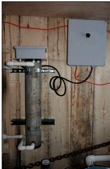
Installation position may also be in a location where it is possible to re-circulate sap from a storage tank through the unit in order to continue treatment if the sap needs to be held in storage for longer than 18 hours. Refrigeration of the sap in addition to UV treatment during long holding times greatly reduces the growth of microorganisms that can consume the sugar contained in the sap.
