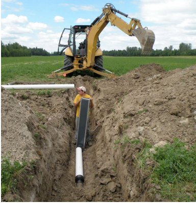
Installing tile drainage in NNY. Photo: Miner Institute
