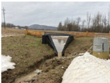
Figure 4, left: Flume capturing surface runoff during snowmelt event on 1/12/18 for undrained field, NNYADP Tile Drainage project, 2017.
